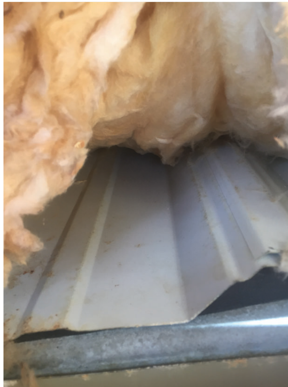
Photo 4 - Inside Roof System - Wet insulation on Lower Metal Sheet
