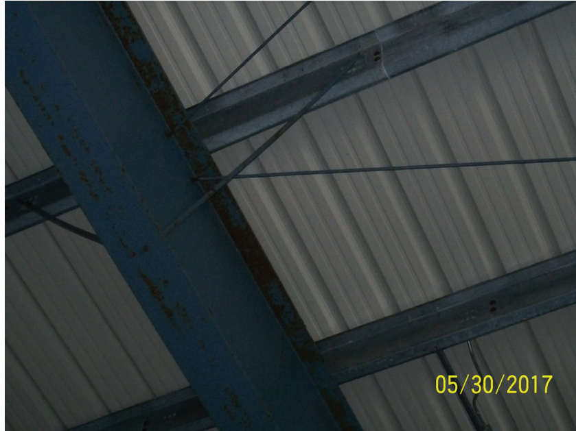
Photo 3 – Rust on main Structure due to Condensation
