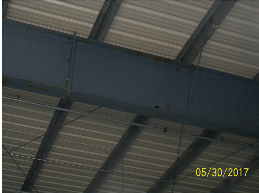
Photo 1 – Rust on Steel Rigid Frame due to Condensation
