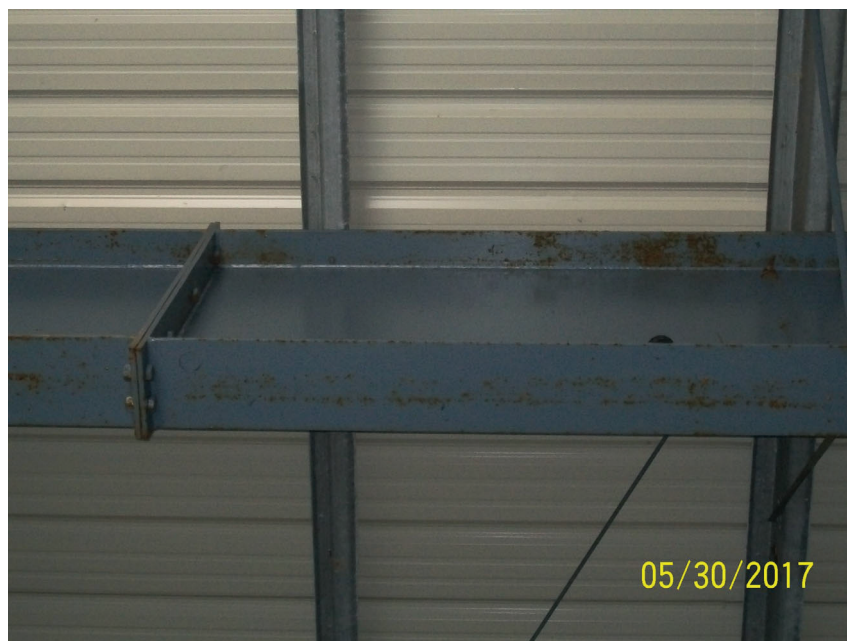
Photo 2 – Rust on Steel Rigid Frame
